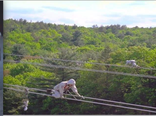
Power line inspection
